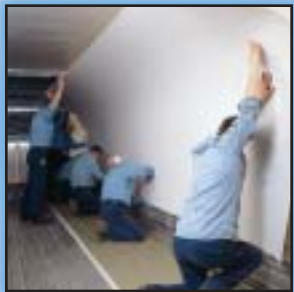
► Liner placed onto trailer wall. Bracing installed to maximize bonding process
